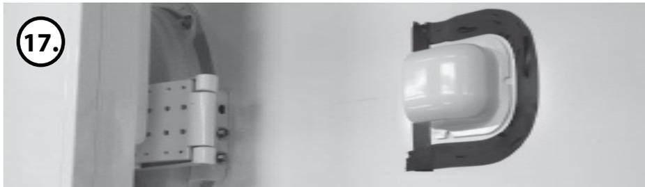
Arrange cable holder in front of (30cm apart from) antenna center by facing open side of cable holder toward projected part of the mounting plate. Then attach friction tape
