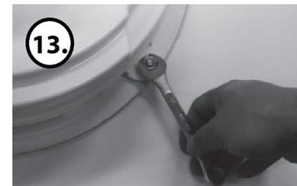
Attach the antenna to the mounting plate
